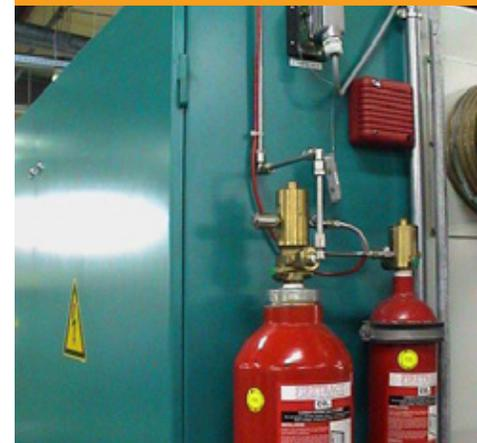
Firetrace offers options such as a manual release and a warning horn, which is triggered by activation of the system.
