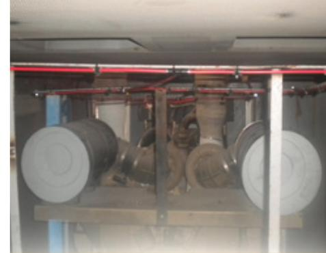
The red Firetrace detection tubing is routed throughout the risk areas, providing fast detection and suppression.
